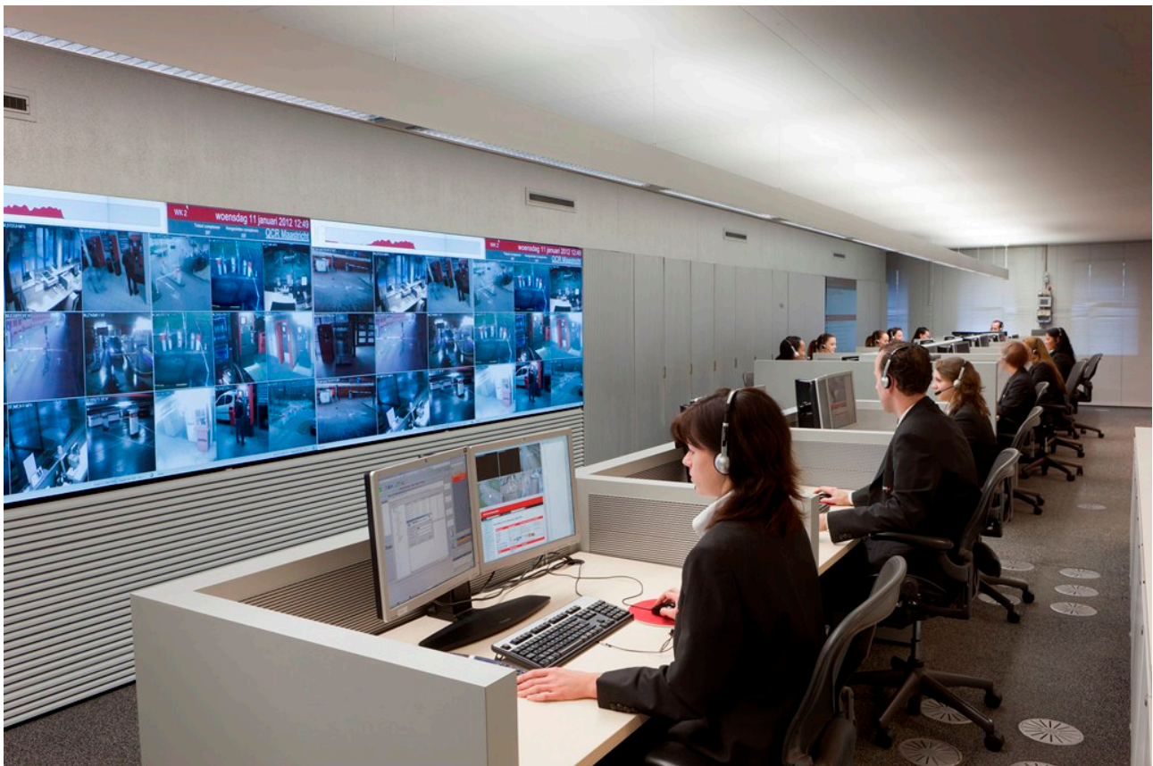
Figure 14: Q-Park Control Room (QCR)
