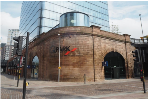
Figure 4: Deansgate North historic facade
